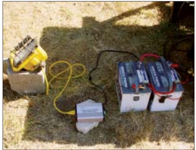
To gauge the effectiveness of the charging system, two deep-cell batteries were wired in parallel; to completely discharge them during the tests, a quartz lamp was used, running off a 300-watt inverter.
